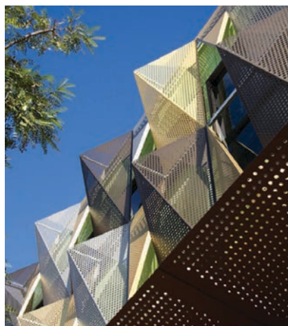
Yanget House, Bunbury, Australia
