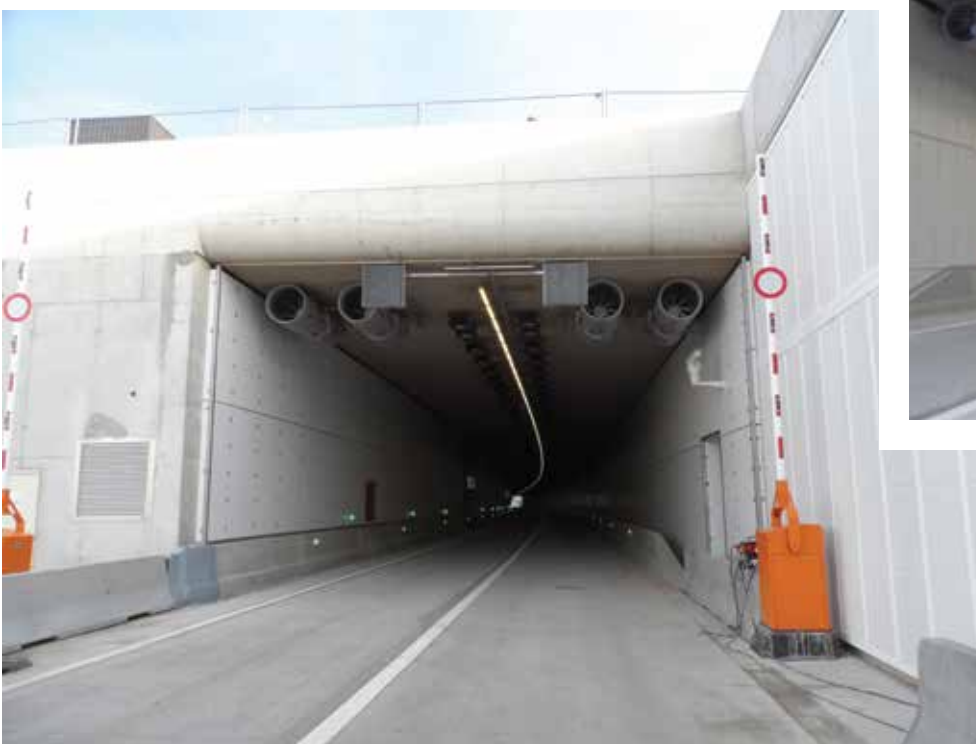
COLT HOLLAND R11 Tunnel, Deurne, Belgium Colt Products: Mechanical induction ventilation with pressurisation systems
