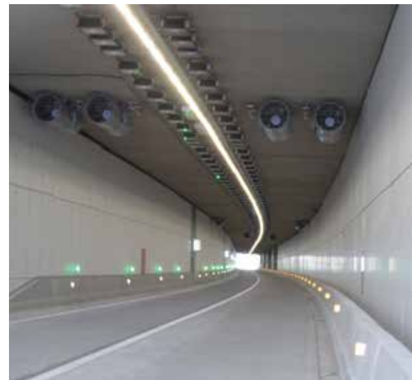
COLT HOLLAND R11 Tunnel, Deurne, Belgium Colt Products: Mechanical induction ventilation with pressurisation systems
